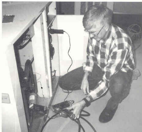
Checking system superheat at the condensing unit.
